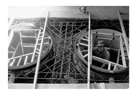
Figure 20-33. Mark Connaughton in the process of constructing underground silos in Southern California for CryoSpan.
