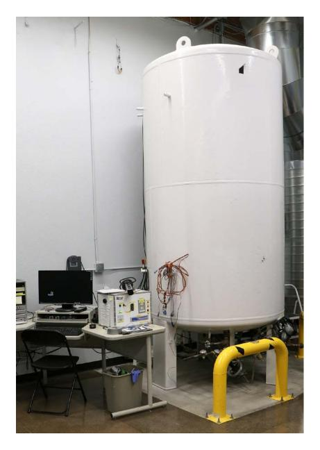
*Figure 20-18. The bulk storage tank for liquid nitrogen in Alcor's patient care bay. Its capacity is 900 gallons.*
