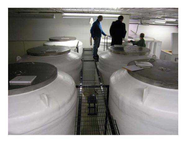
*Figure 20-28. A catwalk allows access to the lids of the cryostats at the Cryonics Institute.*
