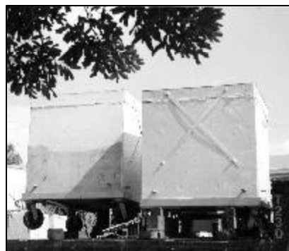
Loading the vaults onto a second flatbed. Right: vault is already loaded and resting securely on its supports. Left: vault is lifted up from underneath by forklift so supports can be placed under it.
